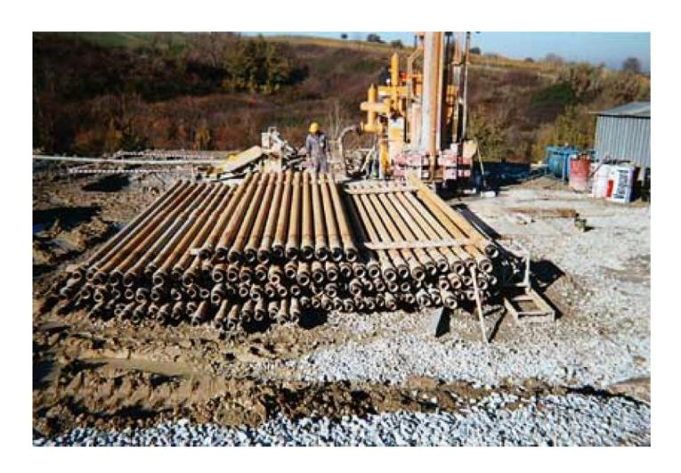
It is a suitable technique for alluvial and rocky soils and to perform medium-tight holes (from 6" (152mm) to 17"1/2 (444mm)) even for high depths.
