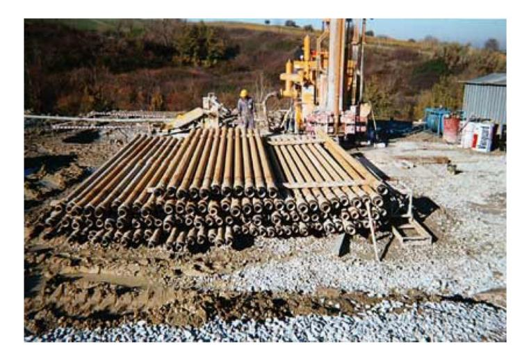
It is a suitable technique for alluvial and rocky soils and to perform mediumtight holes (from 6" (152mm) to 17"1/2 (444mm)) even for high depths.
