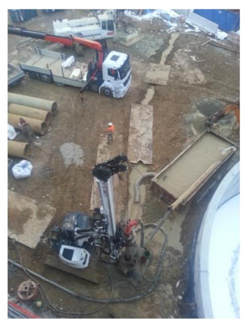
As circulation fluid can be used water or bentonite at low viscosity and density, this can lead some benefits in the final phases of the development of the well, like the draining and the waste disposal.
